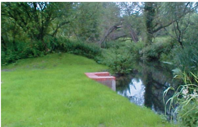
CSO (storm outfall) to River Wey (courtesy Thames Water Utilities Ltd)
