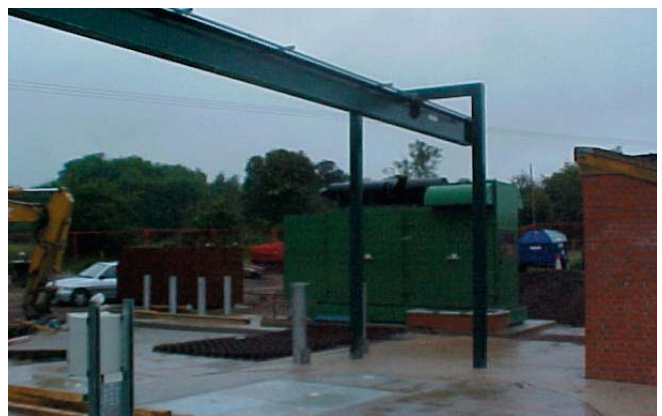
Site under construction (courtesy Thames Water Utilities Ltd)
