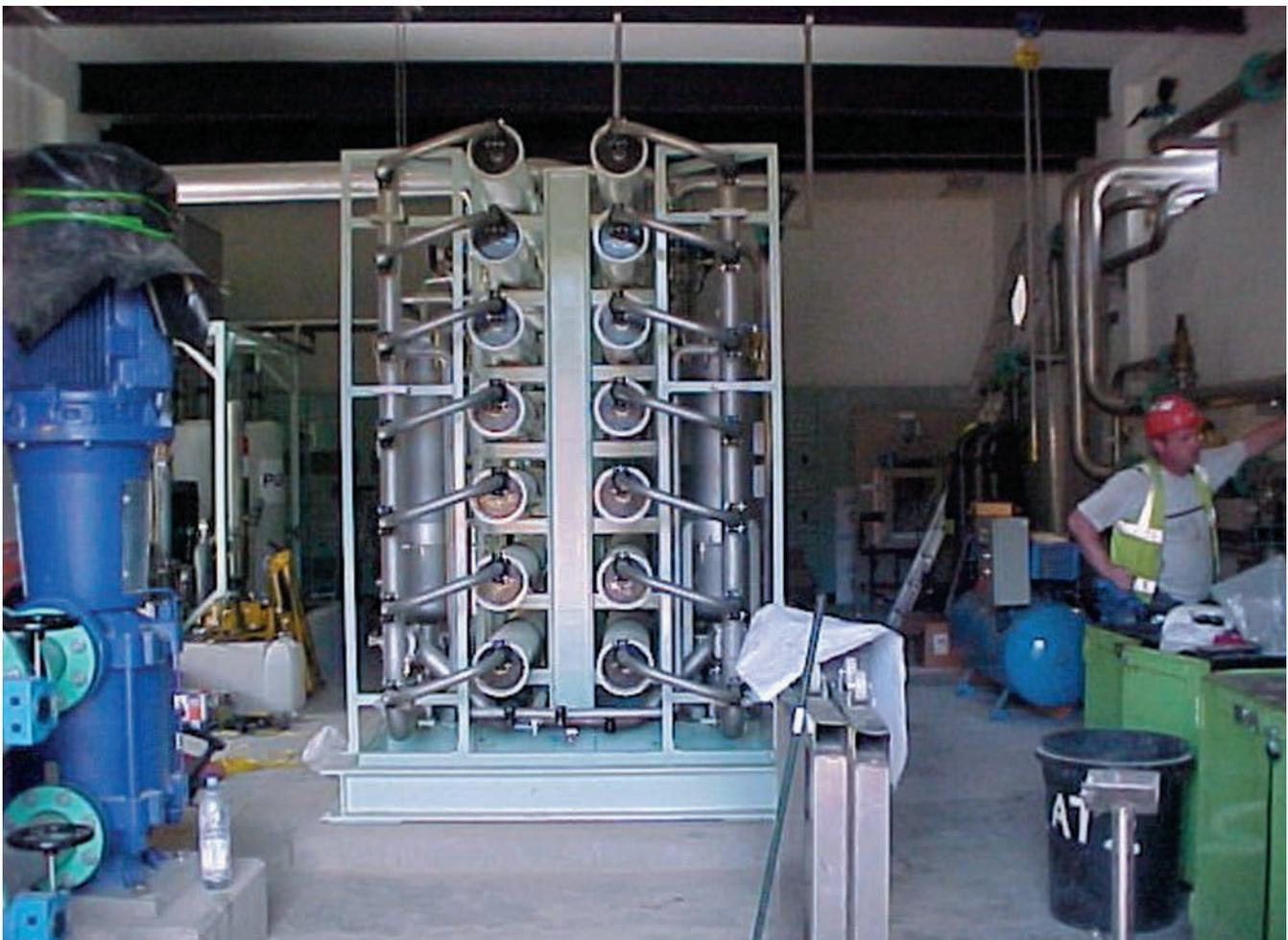
RO Membrane skid in existing pumphouse (courtesy Purac Ltd).
