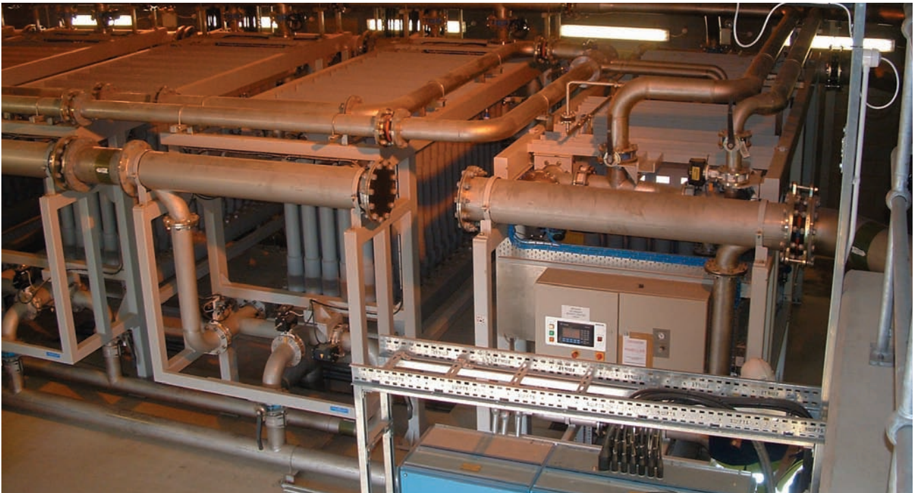
High level Memcor units (Courtesy Memcor & Thames Water)
