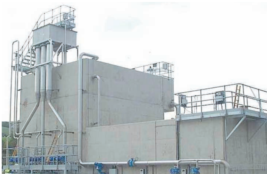
Upgrade works at Chapel-en-le-Frith (courtesy ????)
