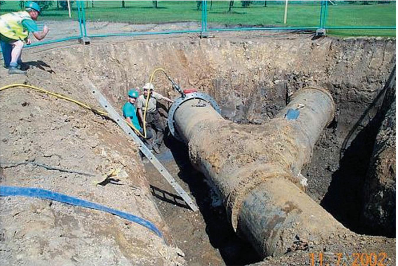
Clear indication of size and scale of rehabilitation work as section of 36" cast iron main is cut out. (courtesy Yorkshire Water Services).
