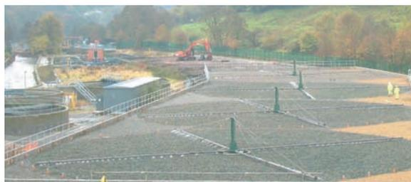
Installation of tile and vent system and installation of filter media at Eastwood
