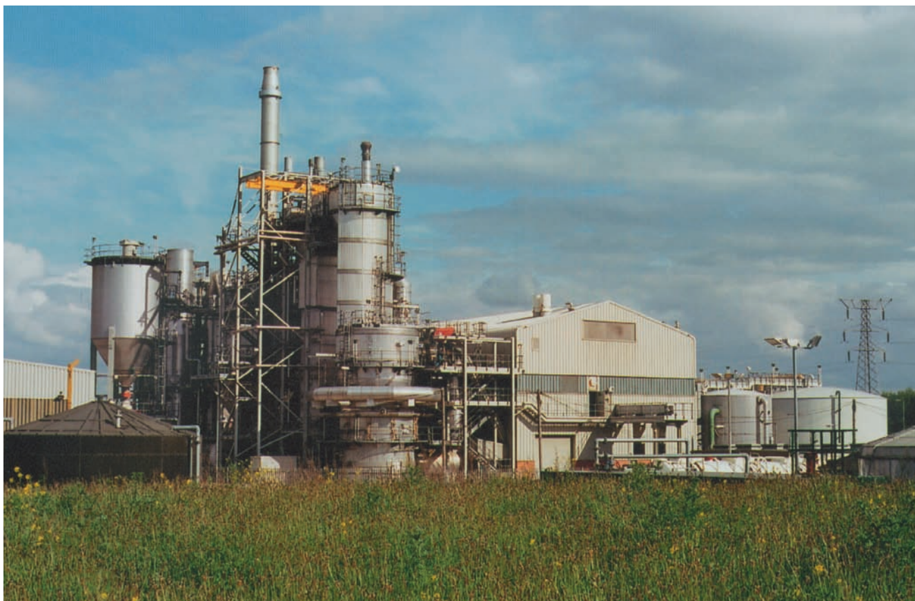
Knostrop Incineration Plant (courtesy Arup)
