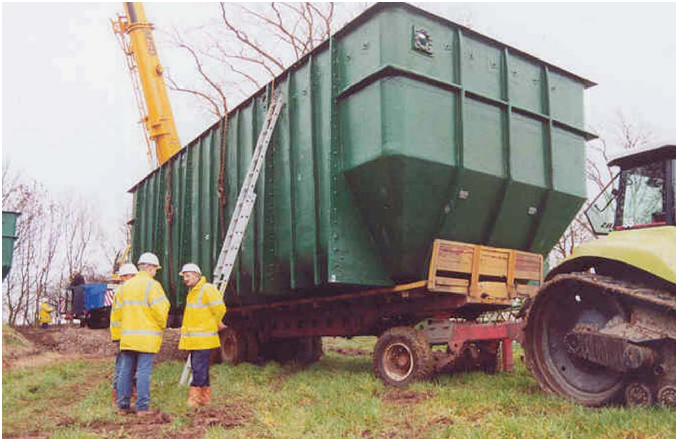
Kirklevington: RBC units fully assembled were towed across fields to site
