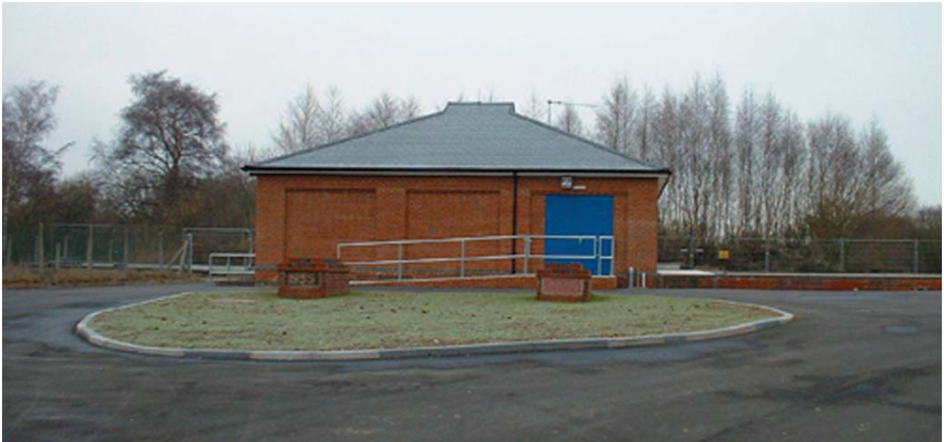
Greywell WTW - New pumphouse
