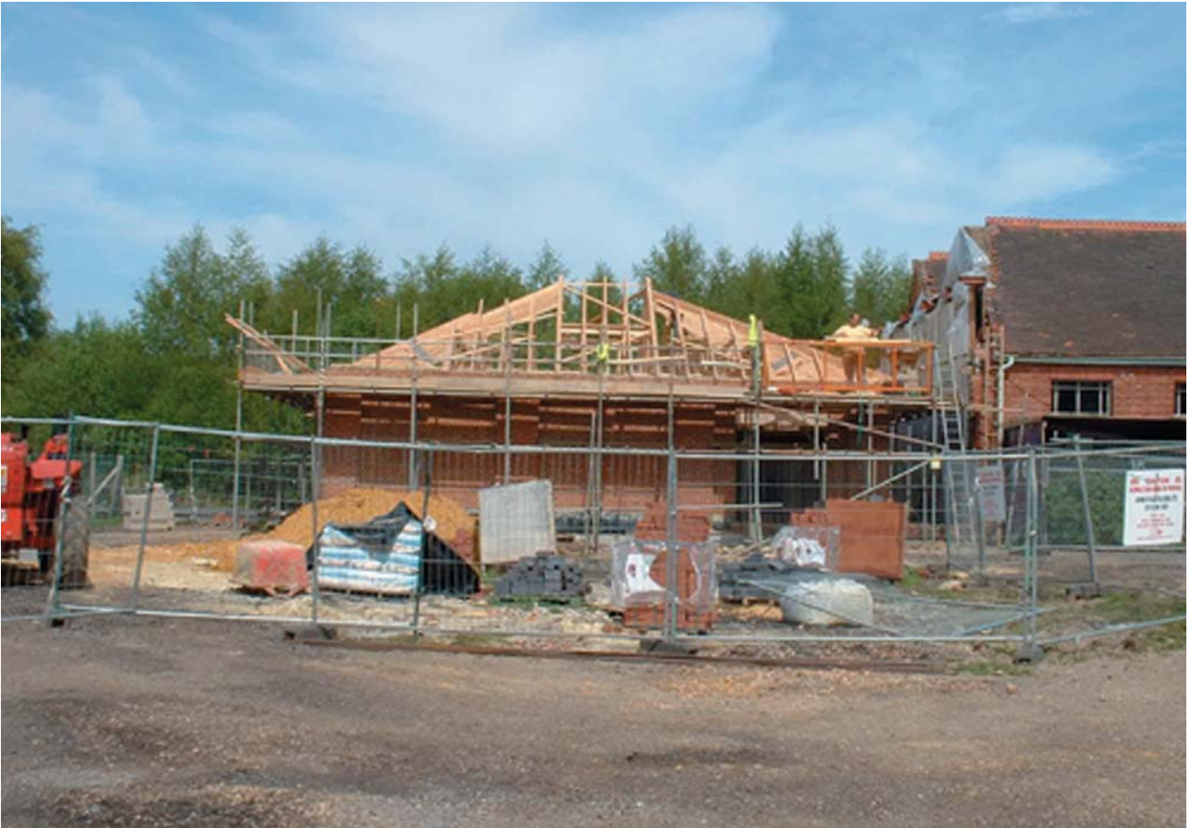
Greywell: Remodelling works in progress
