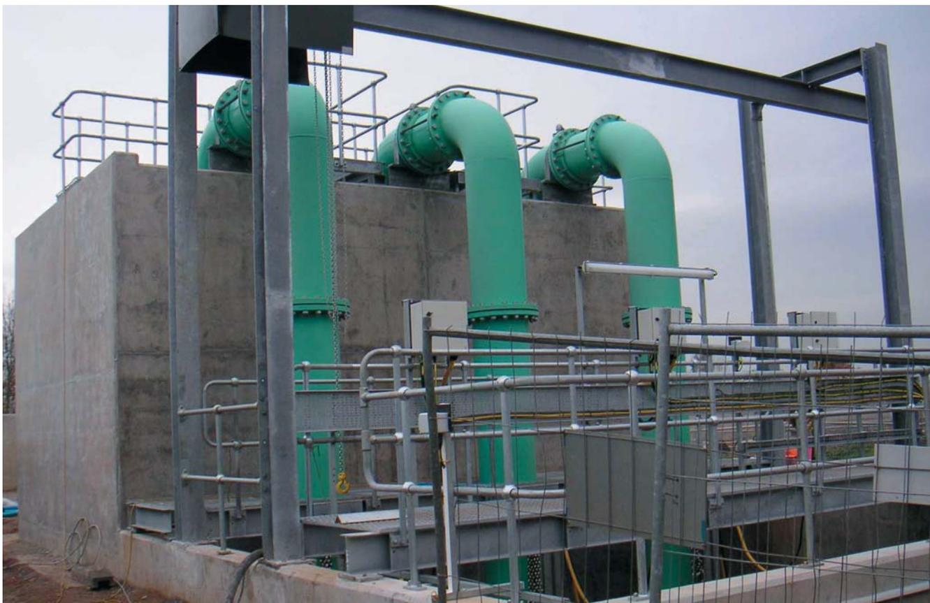
Hartshill: New intermediate pumping station allocates flow between new & existing works
