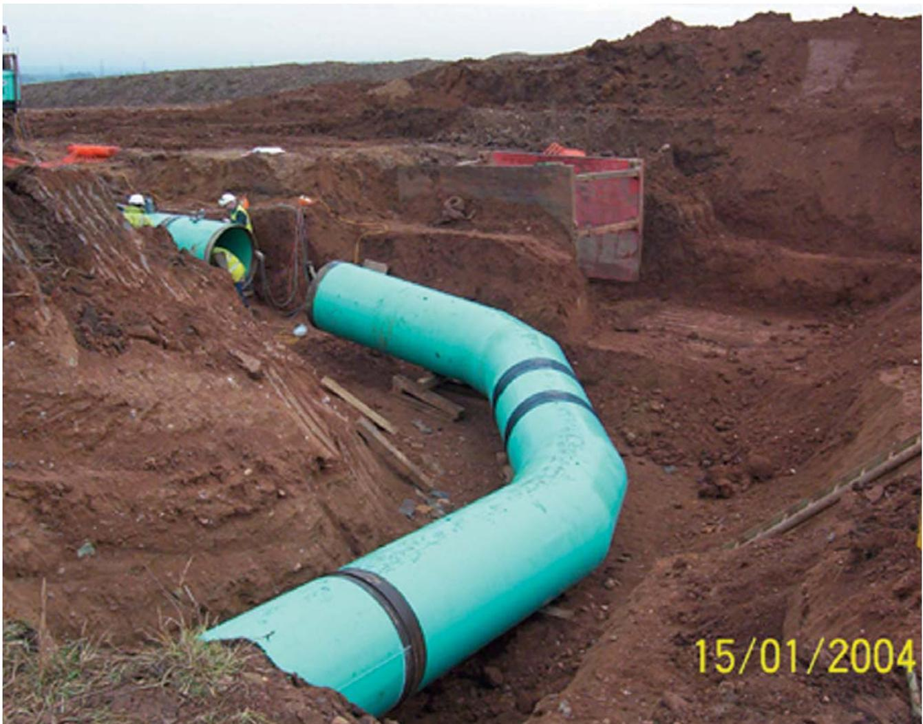
Melbourne WTW: Installation of welded steel pipe
