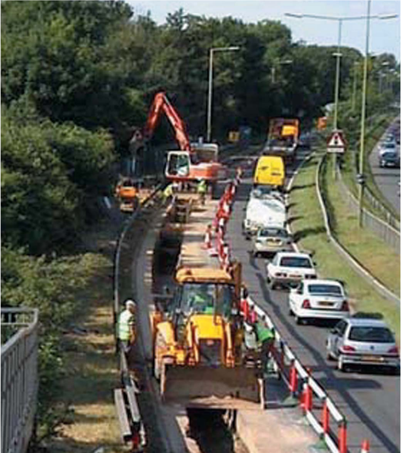
Pipeline construction in southbound carriageway of A10 - June/03
