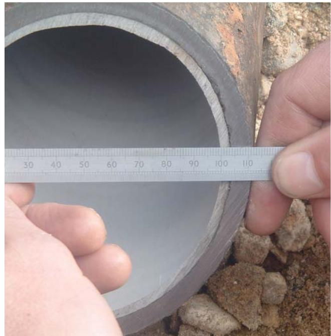
Pipelined with 3mm of semi structural material
