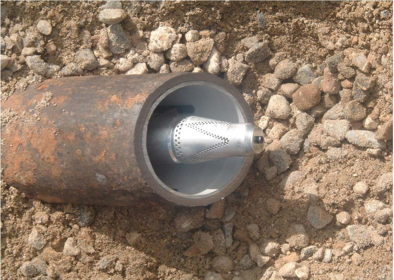
Semi structural resin pipe lining - photo shows spray head & lined pipe
