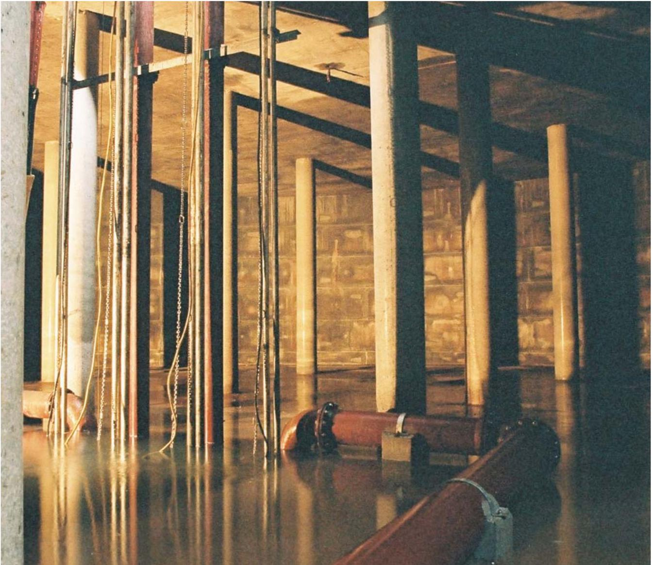
Internal view of large storage tank - 2350m<sup>3</sup> at Taunton Rd PS under construction
