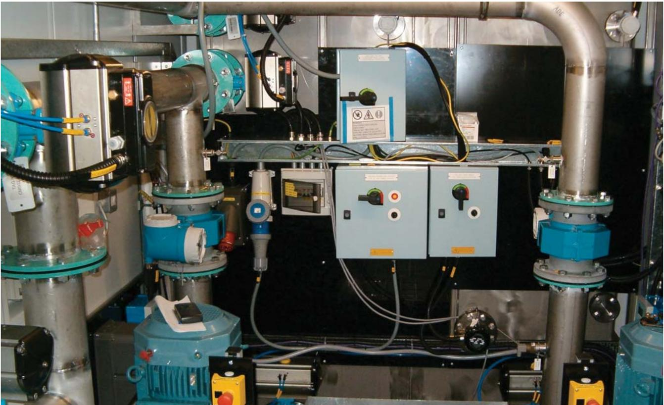
Inside a container the Emergency Packaged Water Treatment plant being fitted out
