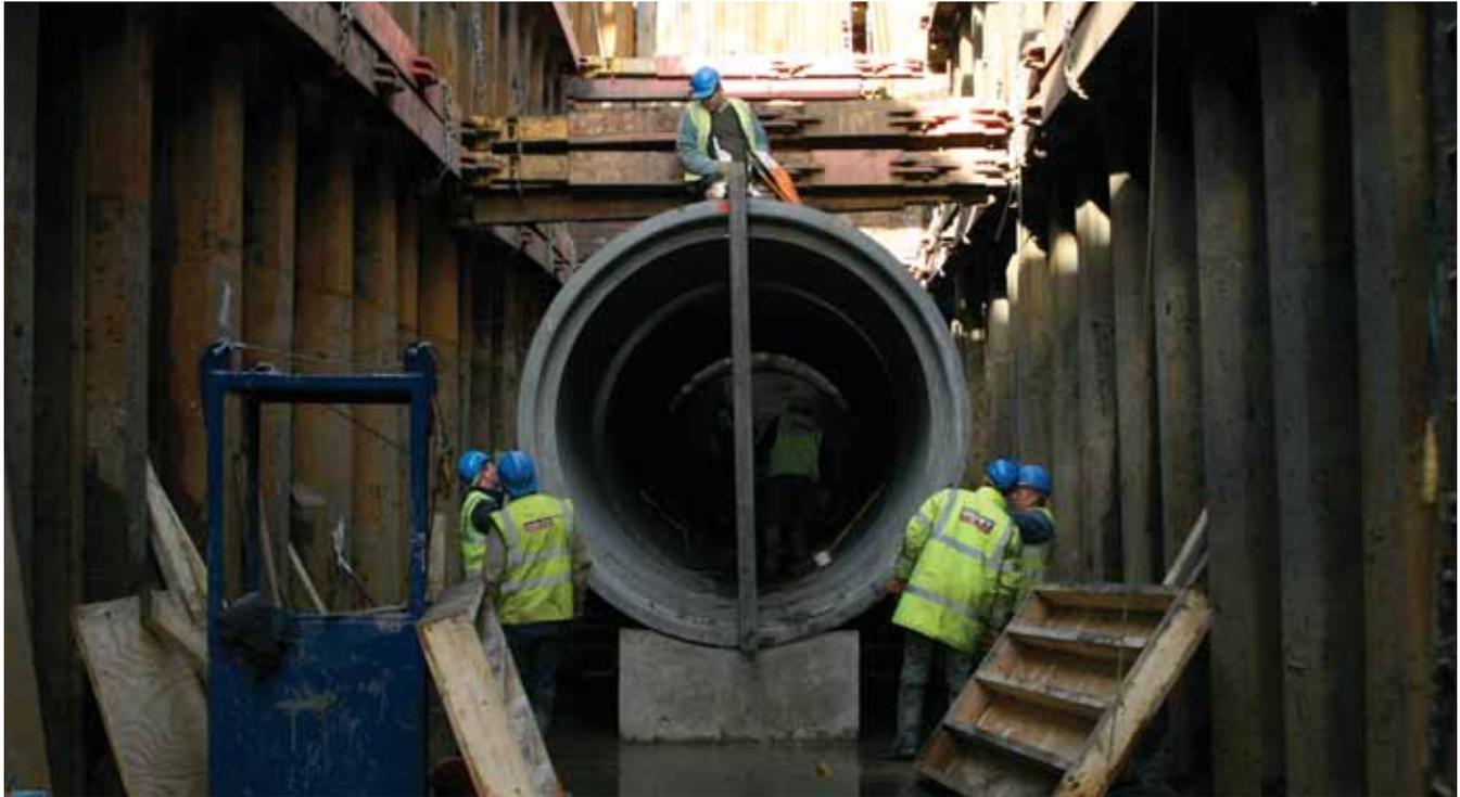
Knothrop Sewer: Placing of concrete pipes - note man standing upright inside pipe
