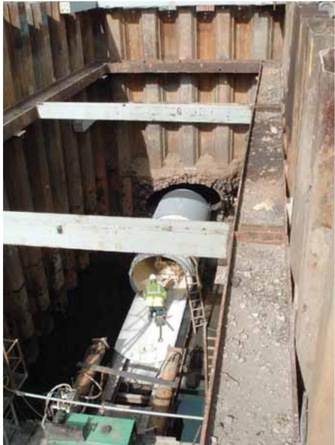
Shield and first pipe prior to jacking within the sewer courtesy: MWH
