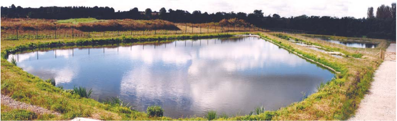
Part of the Ecological Wastewater Treatment System
