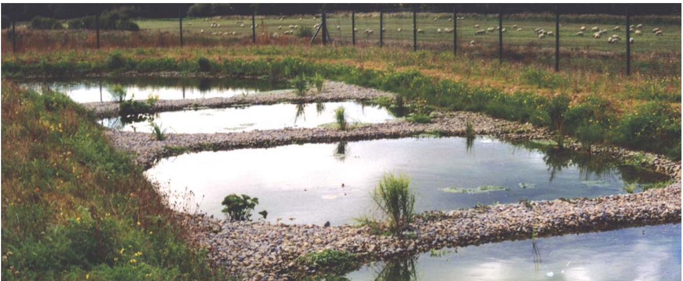
Part of the Ecological Wastewater Treatment System
