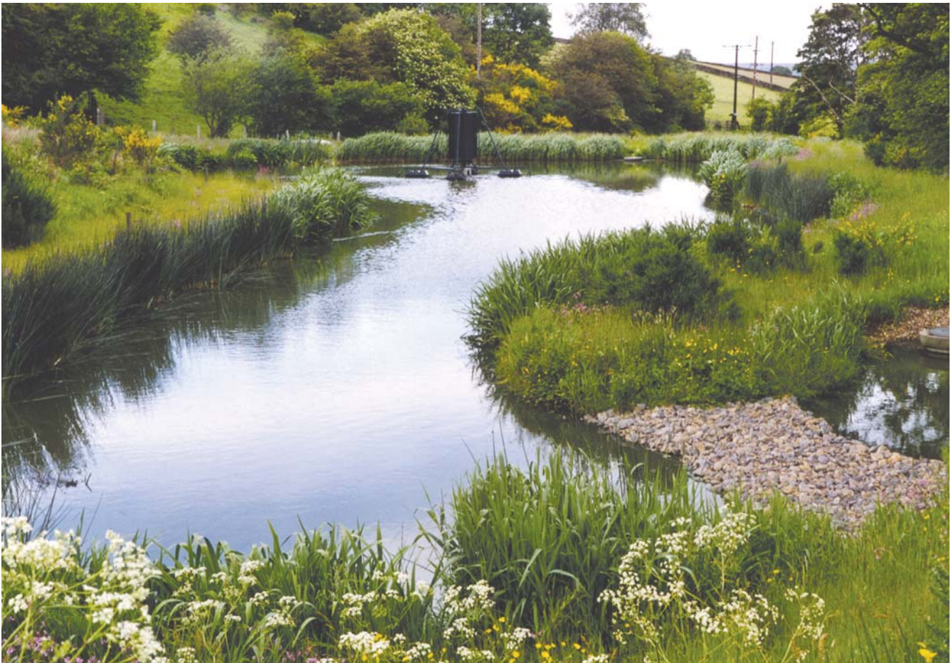
Part of the Ecological Wastewater Treatment System
