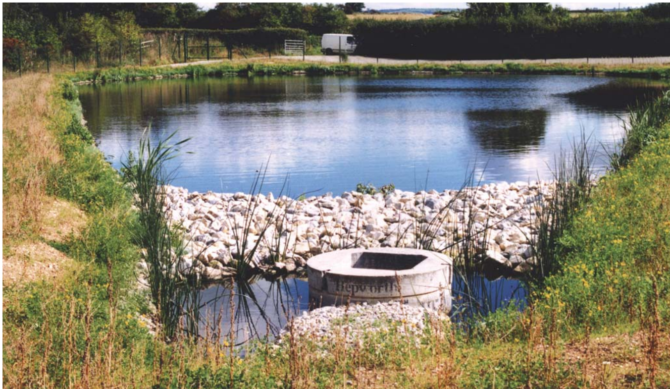
Photo shows one of the ecological ponds in the wastewater treatment system
