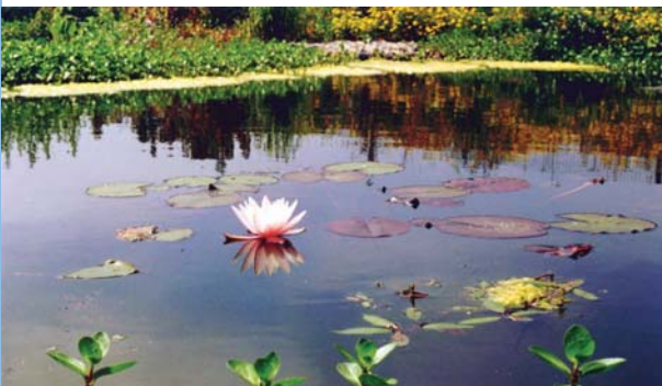
Final rock filter & pond in the ICE award winning Scrayingham Ecological Wastewater Treatment System
