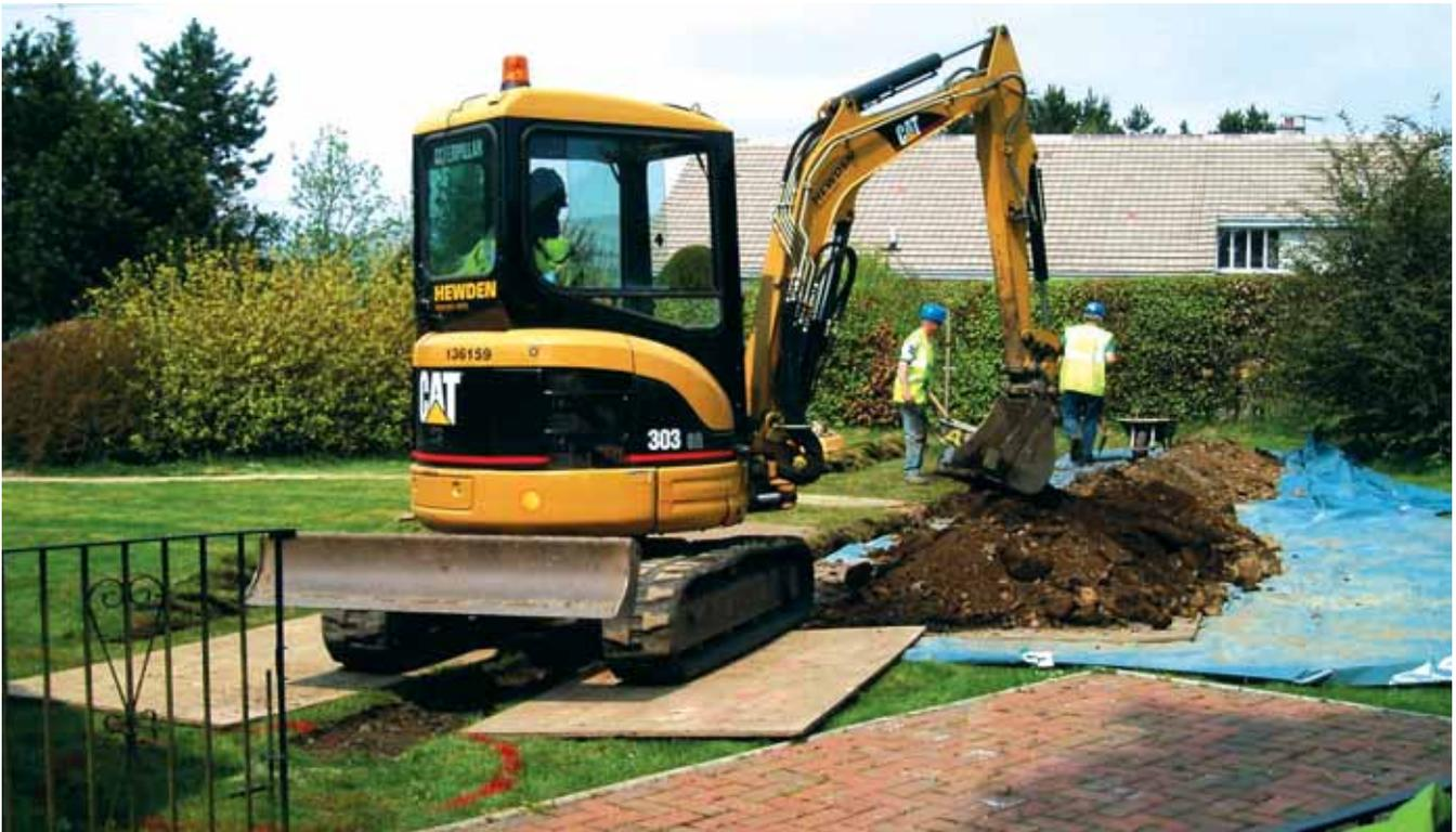
Drum: Vacuum sewerage installation
