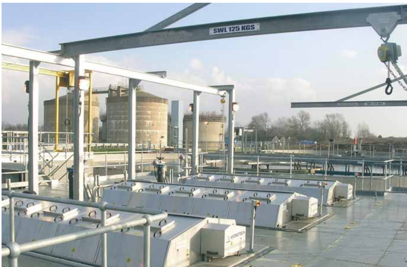
Slough STW: Discfilters being installed
