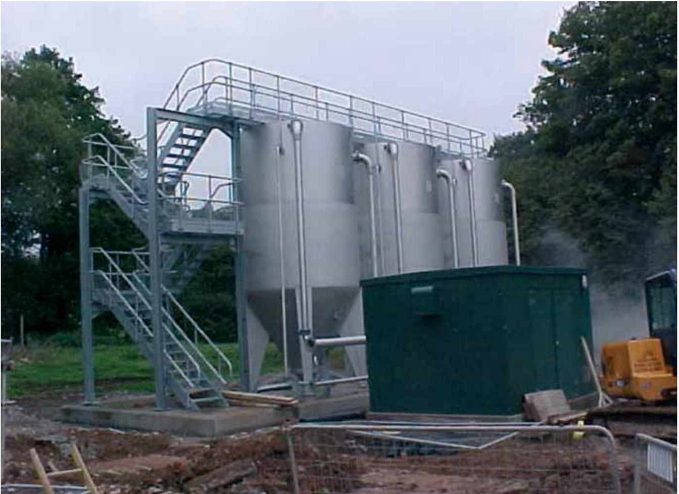
Chew Stoke: New tertiary sand filters under construction
