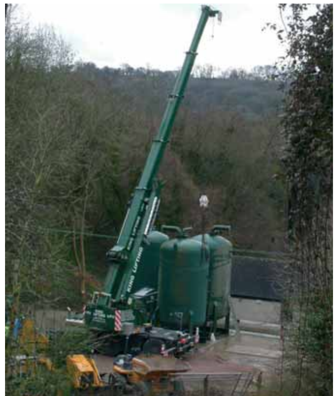
Installing GAC vessels
