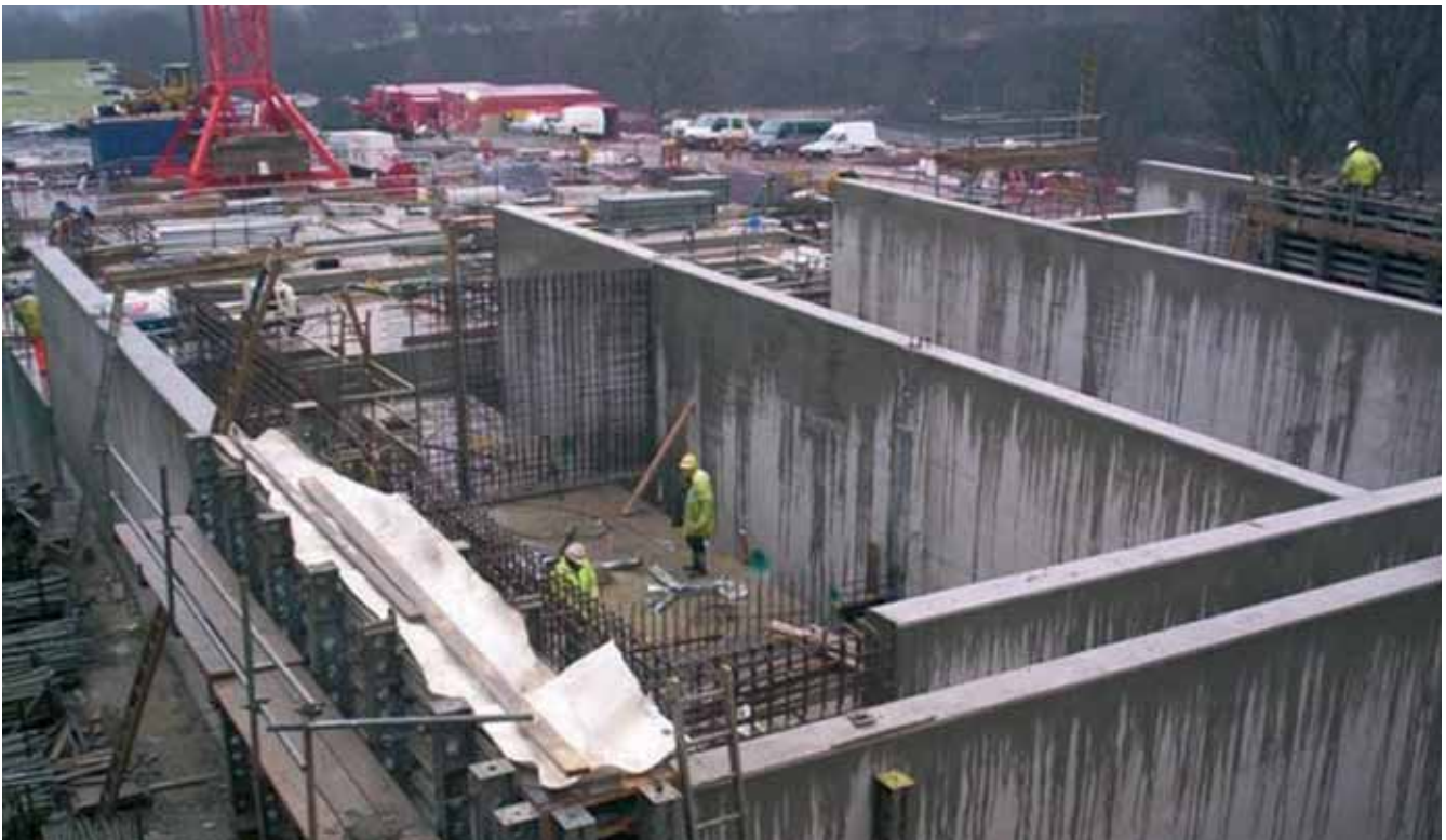
Construction of contact tank + manganese contactors
