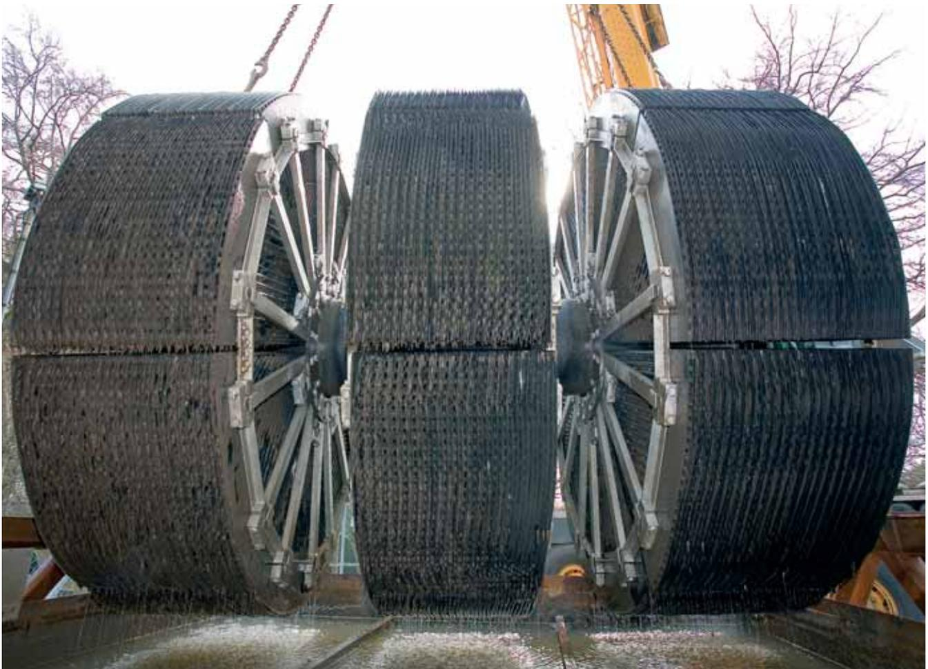
Wortley East: Lifting the new Rotating Biological Contactor into place
