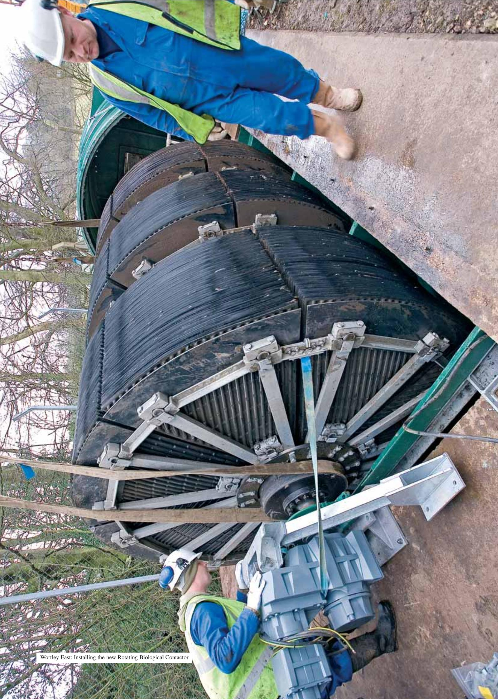
Wortley East: Installing the new Rotating Biological Contactor
