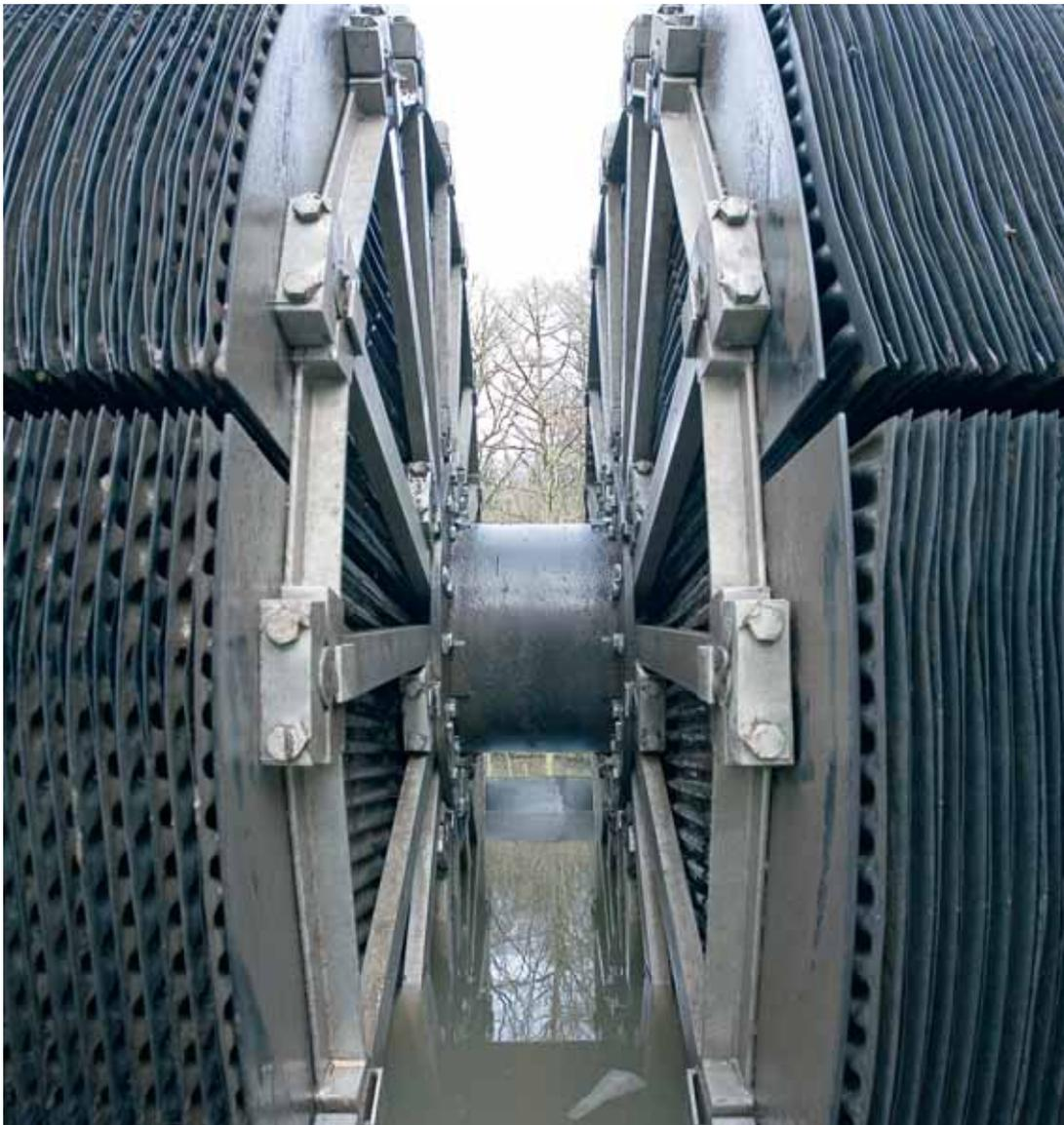
Wortley East: Rotating Biological Contactor in temporary tank preparing for installation
