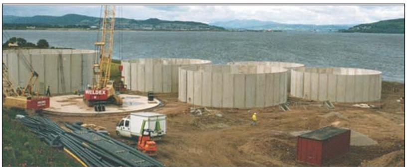
*Aqua-Tanks* being installed at Inverness – the concrete panels are held together by means of a high-yield steel tendon system
