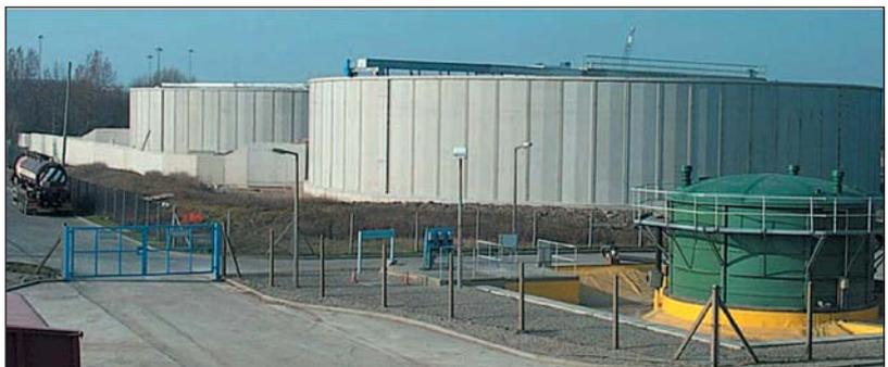
Two 45m diameter x 8m high stormtanks for Wessex Water at Bristol Wastewater Treatment Works
