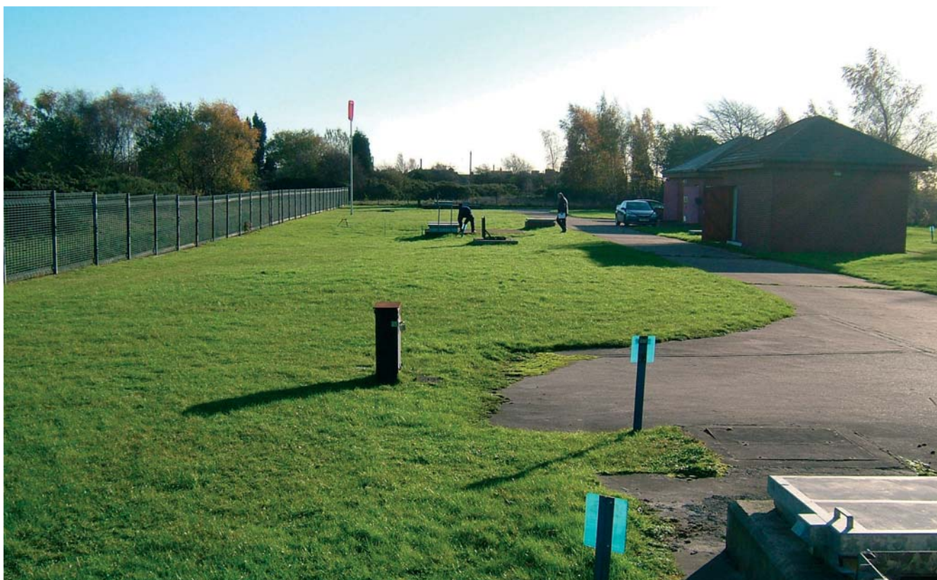
Eggborough WTW. One of the many WTW being made redundant as a result of rationalisation
