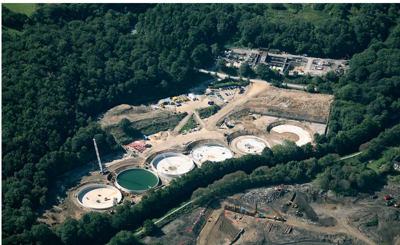
Yorks FFD: Primary tank construction underway upgraded inlet works in background
