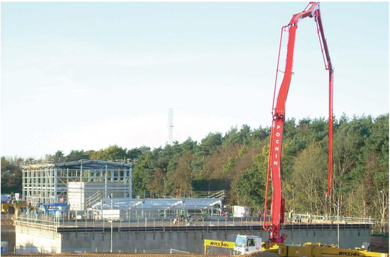
63 metre concrete pump pouring reservoir roof
