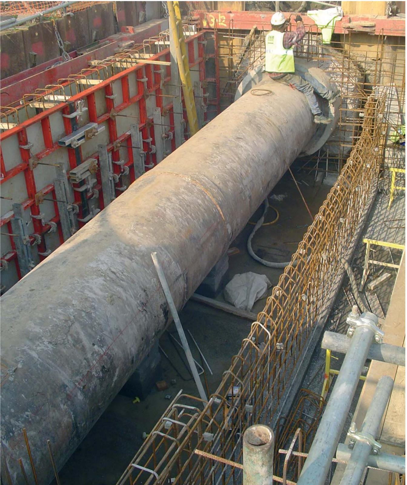
*Fluming existing flows through new CSO chamber during construction*
