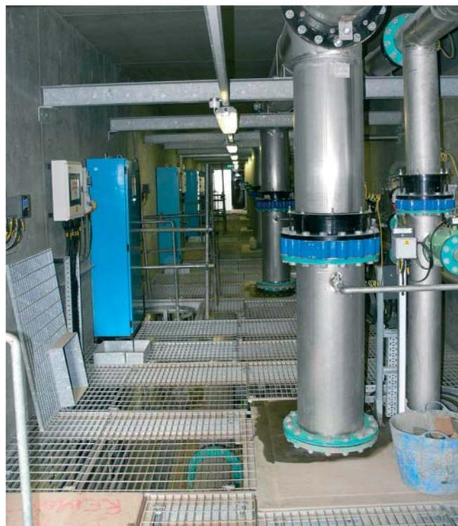
*Backwash and eductor pipework in GAC Plant Gallery courtesy MWH*
