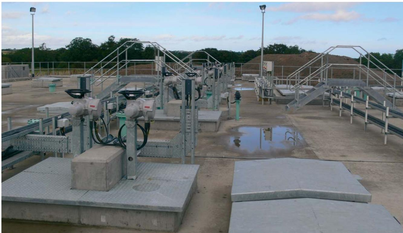
GAC Plant roofline showing actuated penstocks, access covers and instrumentation
