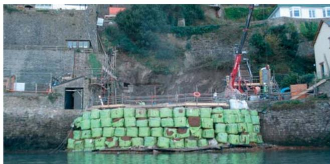
*Temporary cofferdam at pumping station site Photos courtesy Paul Hunt of Black & Veatch Construction of pumping station shaft*
