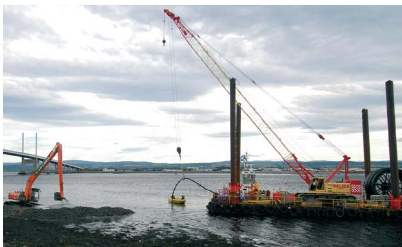
*Commercial Marine & Piling installing, trenching and backfilling sewage pumping main across the Beaully Firth in water currents up to 7 knots. 2007*
