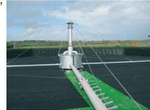
Effluent is applied to the media surface at up to 48 lt/sec by one of our all stainless tubular arm type HYCOVER rotary distributor units fitted with an electro/pneumatic drive unit.
