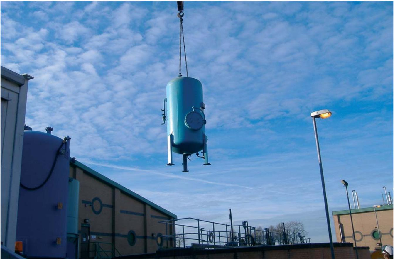
*DAF Saturator Vessel being offloaded at site*
