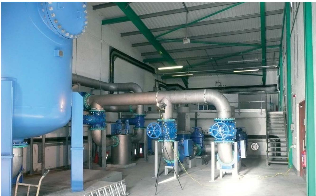
*DAF Saturator vessel and new recycle pumps*
