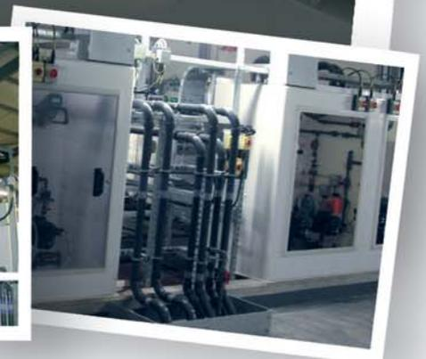
Under a contract awarded by Veolia Water Solutions and Technology (VWS), Gee & Company has installed the bulk of the dosing equipment for the Actiflo™ clarification process to treat abstracted water as part of Thames Water's upgrade of Fobney Advanced WTW in Reading.
