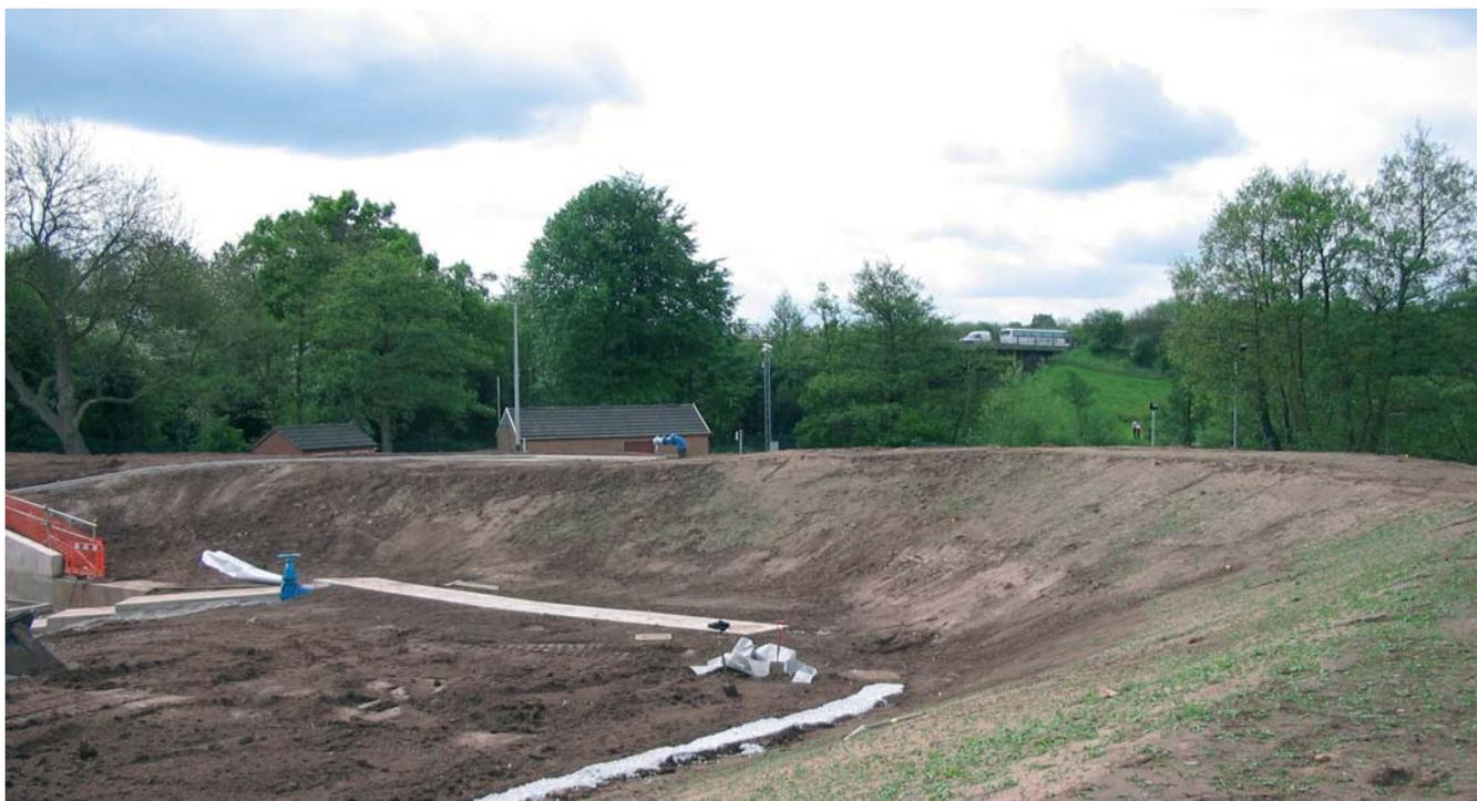
*Intake pumping station in Chester, which draws water from the River Dee, with a view of flood defence (earth embankment) under construction. photo courtesy Mouchel*
