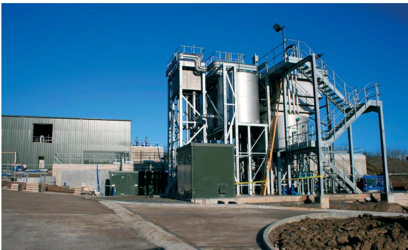
*Poaka Beck WTW Photo shows Lamella Thickeners installed*
