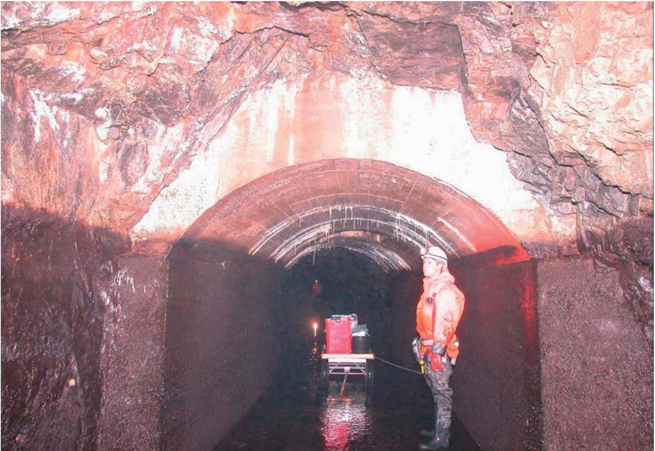
*Aqueduct shows change of construction from unsupported rock to concrete lined tunnel*
