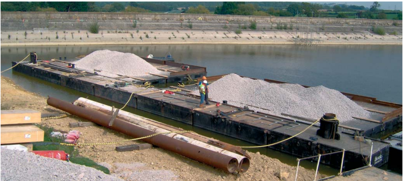
Work on the Sutton Bingham dam near Yeovil
