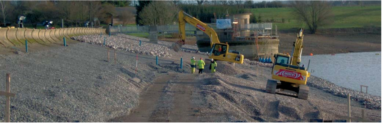
Work on the Sutton Bingham Dam near Yeovil
