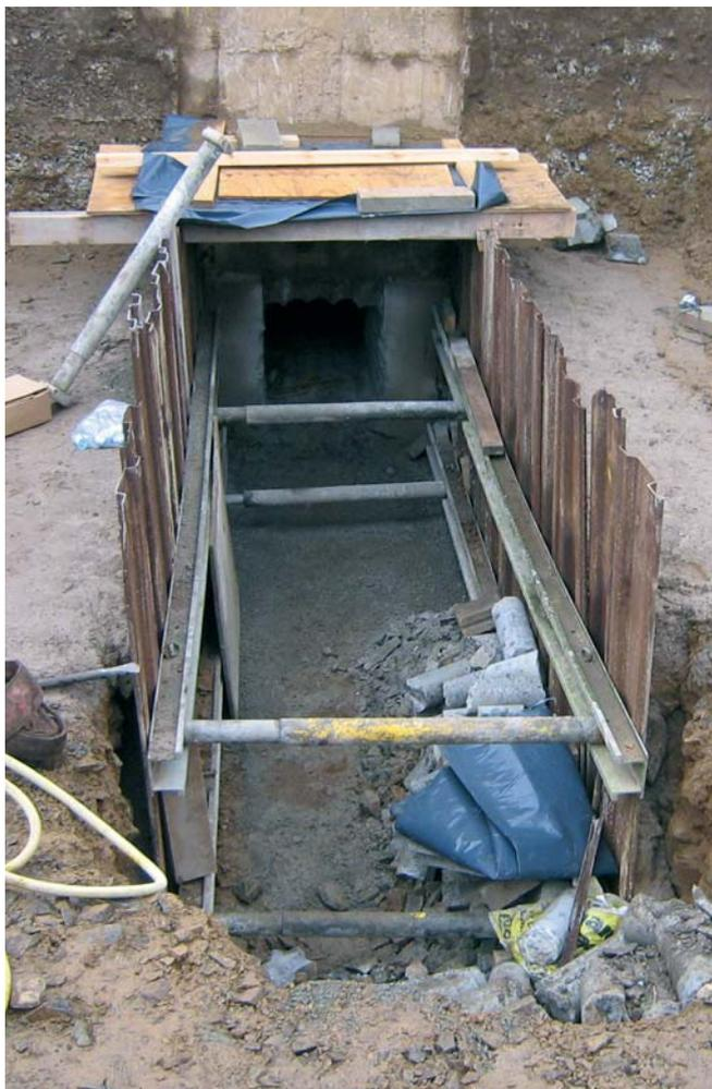
Photograph showing the cutting through the 1.8m thick walls of Tank 1 to install new outlet pipe work
