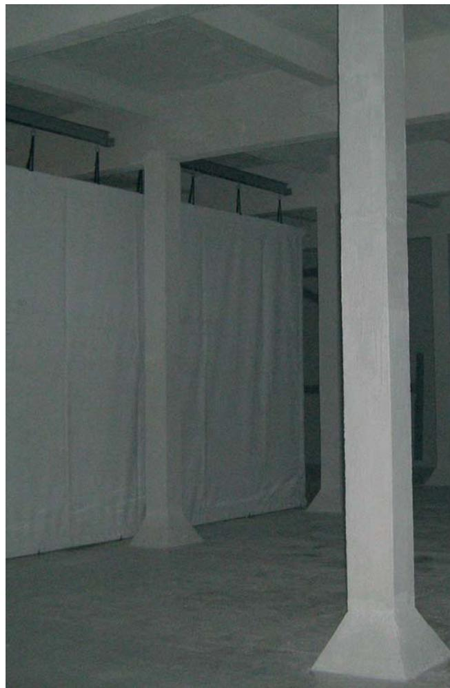
Photograph showing completed works in Tank 1, with sealant coating applied and baffle curtains installed
