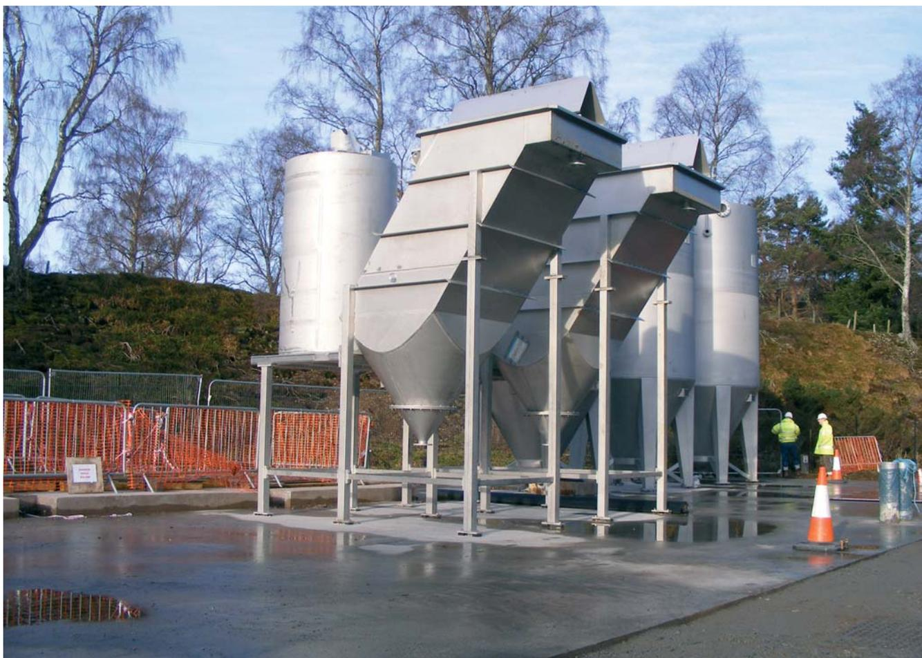
*Dynasand filters and Lamella clarifiers before the erection of the new building*
