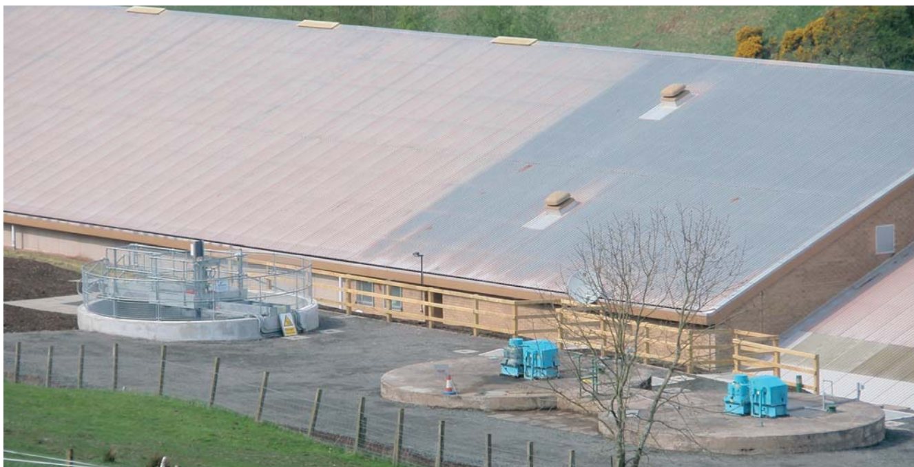
New Sludge Thickener (constructed from precast construction) adjacent to the existing cast insitu with roof thickeners
