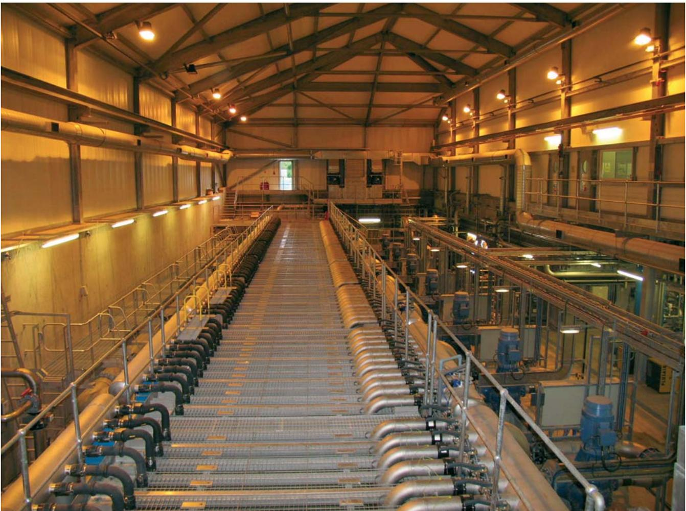
*Invercannie WTW Memcor Membrane plant – Membranes were upgraded for a type compatible with colour removal*
