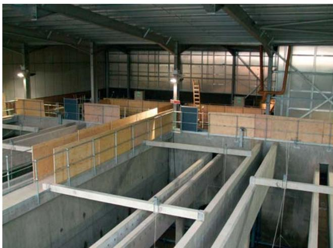
*Extension to Mannofield WTW (right) and Internal view with the 2 (No.) new clarifiers in the foreground and the 2 (No.) new RGSFs in the background (left)*
