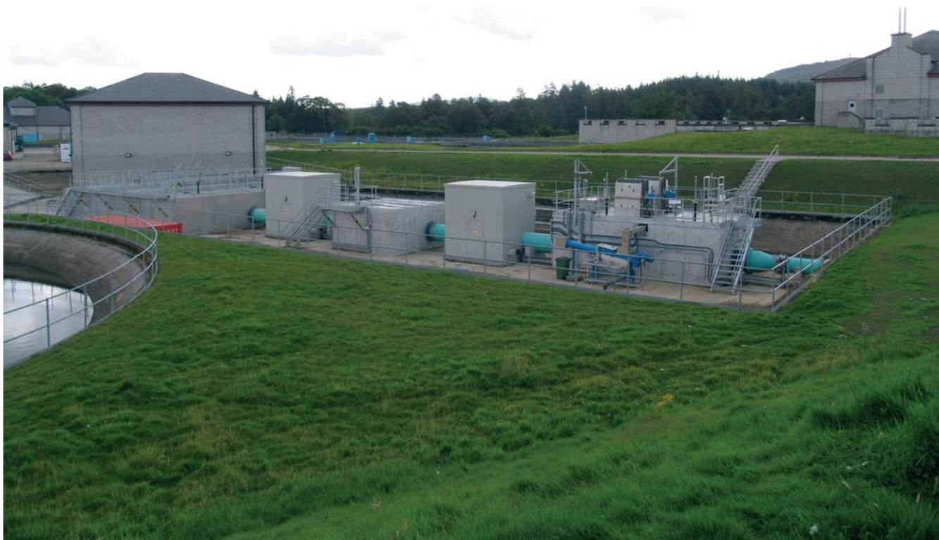
*Invercannie WTW - New inlet works which includes a screening chamber, chemical dosing, flocculation tank and a new chemical building. These were all contained within an existing slow sand filter which was taken out of service early to accommodate the new inlet works*
