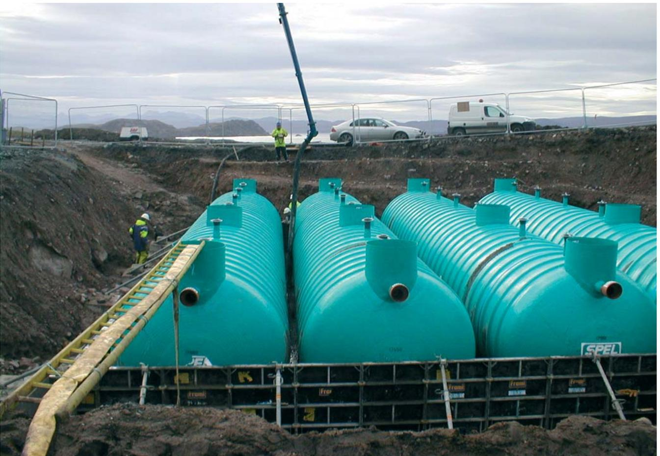
*Placing concrete surround to WWTW tanks*
