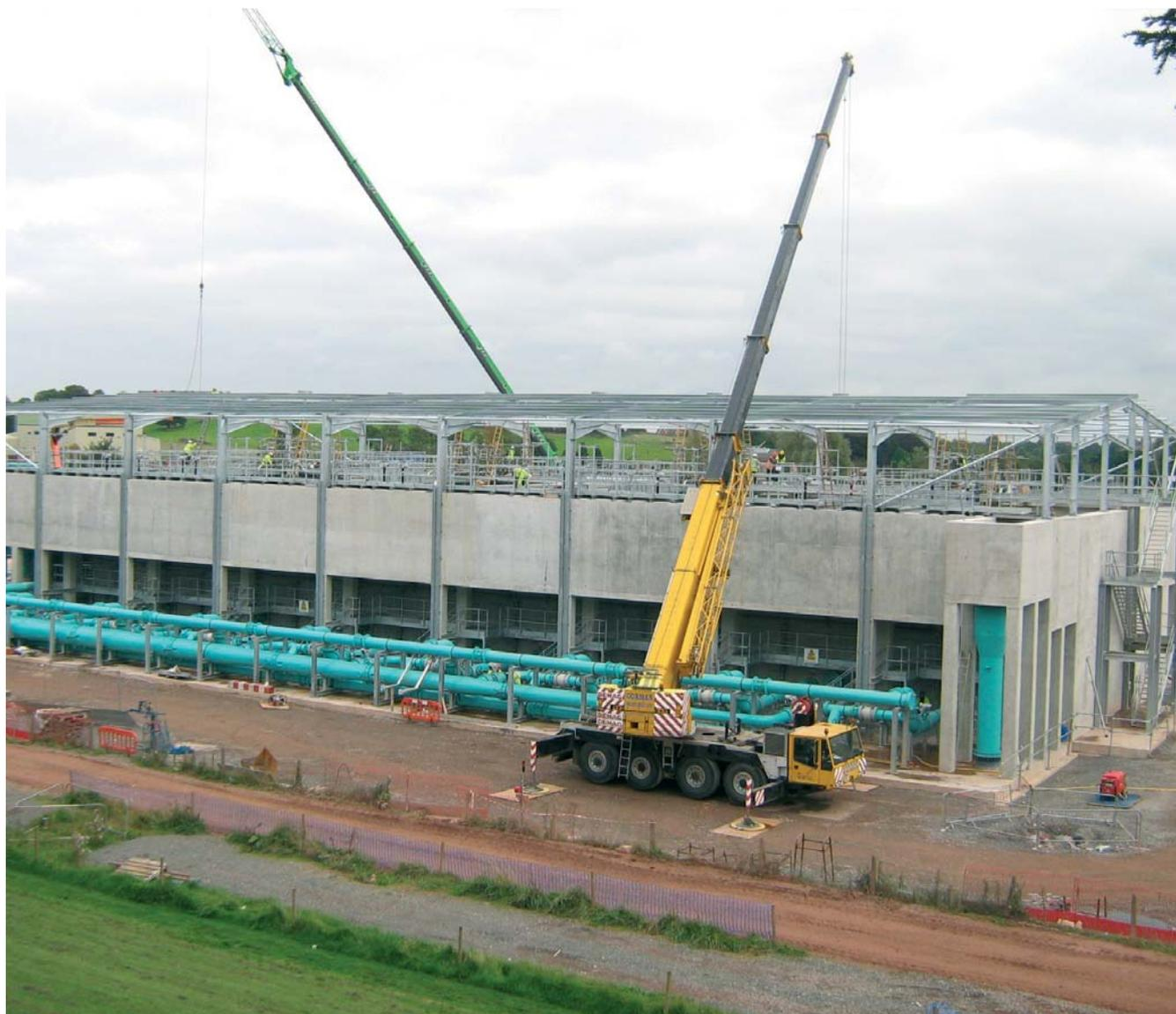
Construction of Portal Frame steelwork around GAC Cell Structure and process pipework
