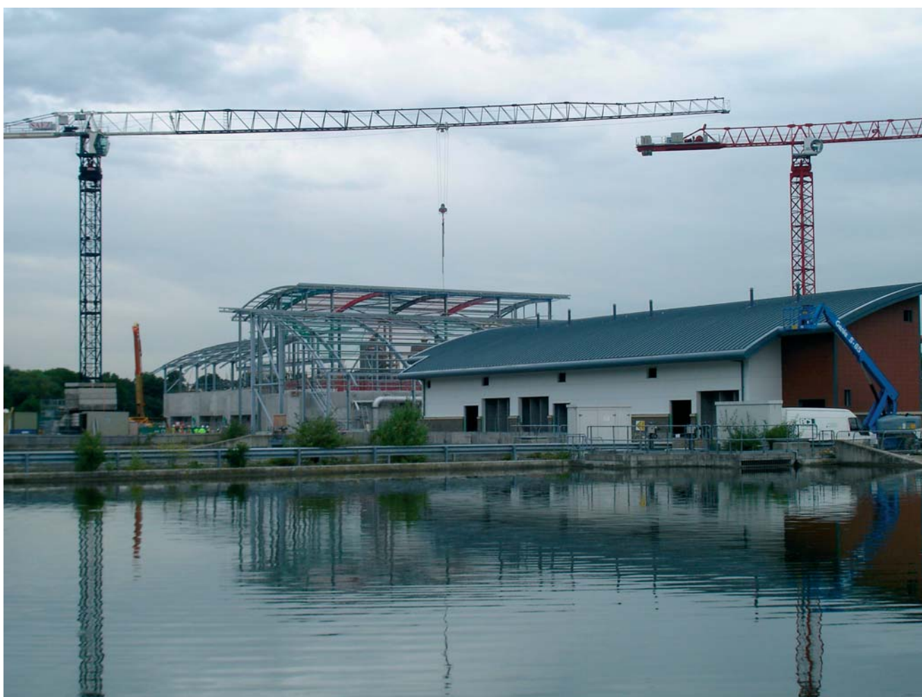
Hornsey WTW under construction
