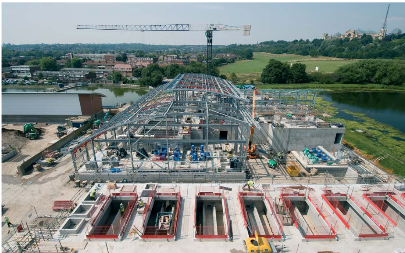
Hornsey WTW under construction
