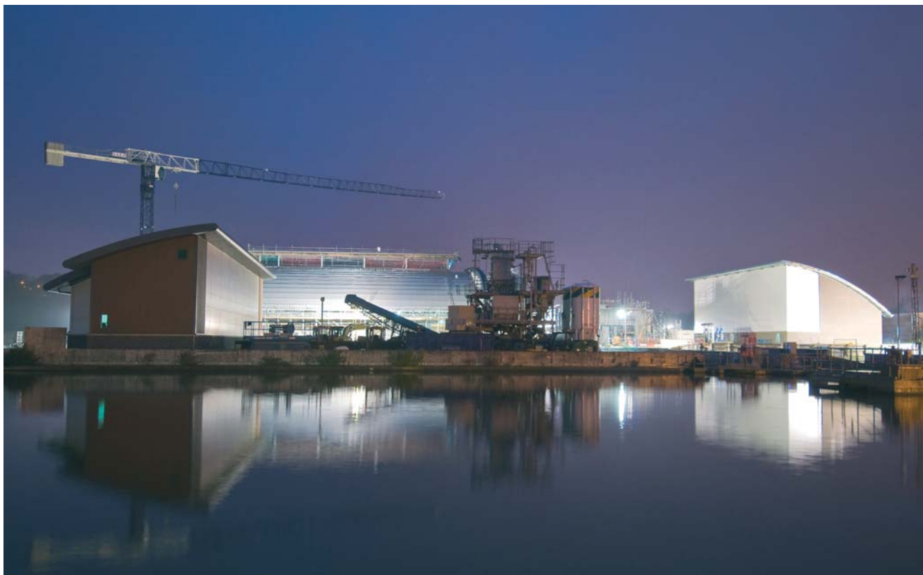
Hornsey WTW under construction
