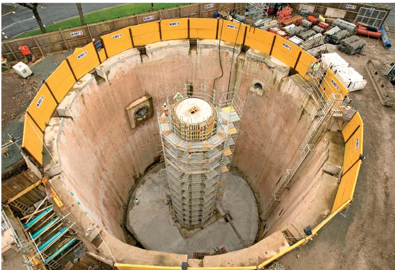
Detention Tank Showing Vacuum Flushing Column Construction
