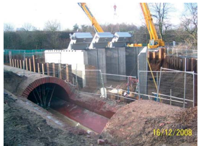
Princess Parkway Screening Chamber and Existing Brick Arch overflow culvert
