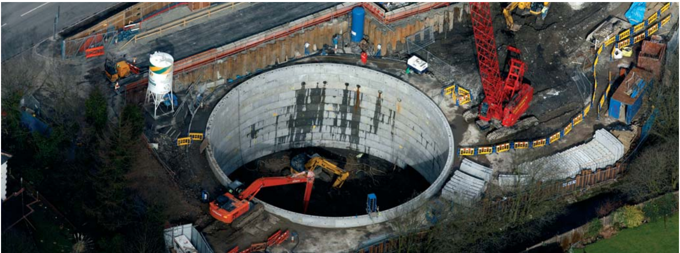
Rossendale Detention Tank
