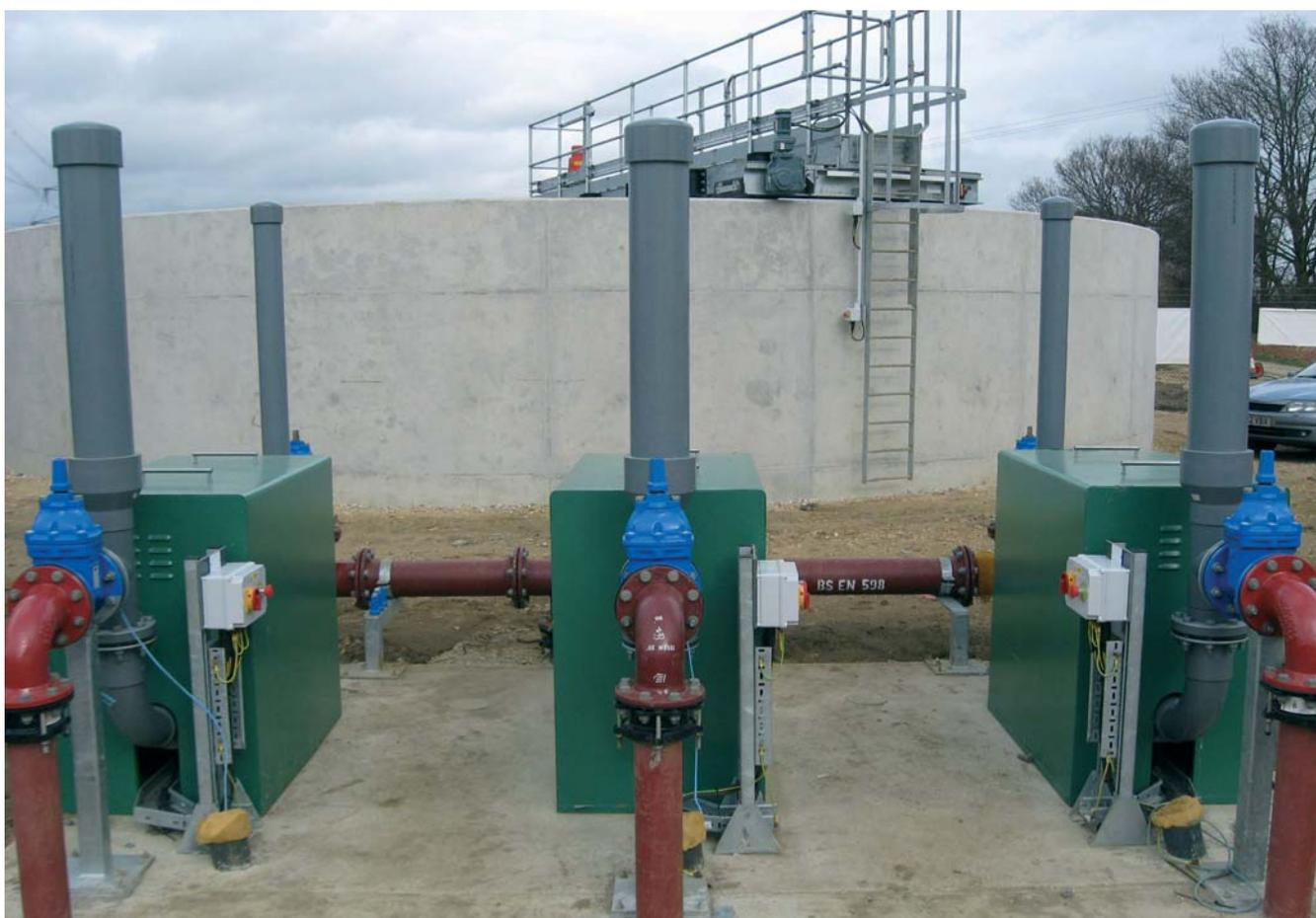
Primary balance tank with scraper bridge plus primary balance tank pumps
