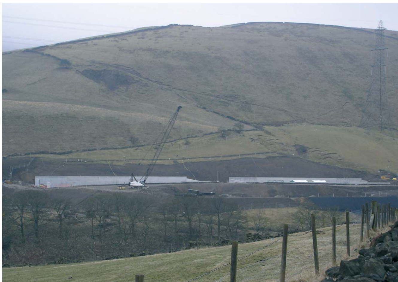
View of settlement lagoons under construction
