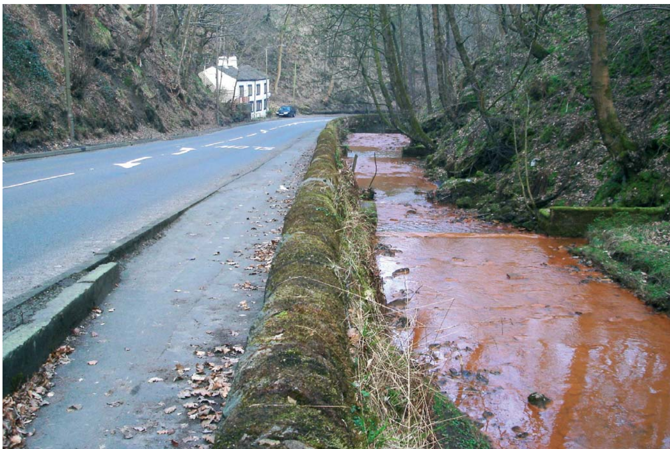
Photograph of ochre staining of Midgelden Brook
