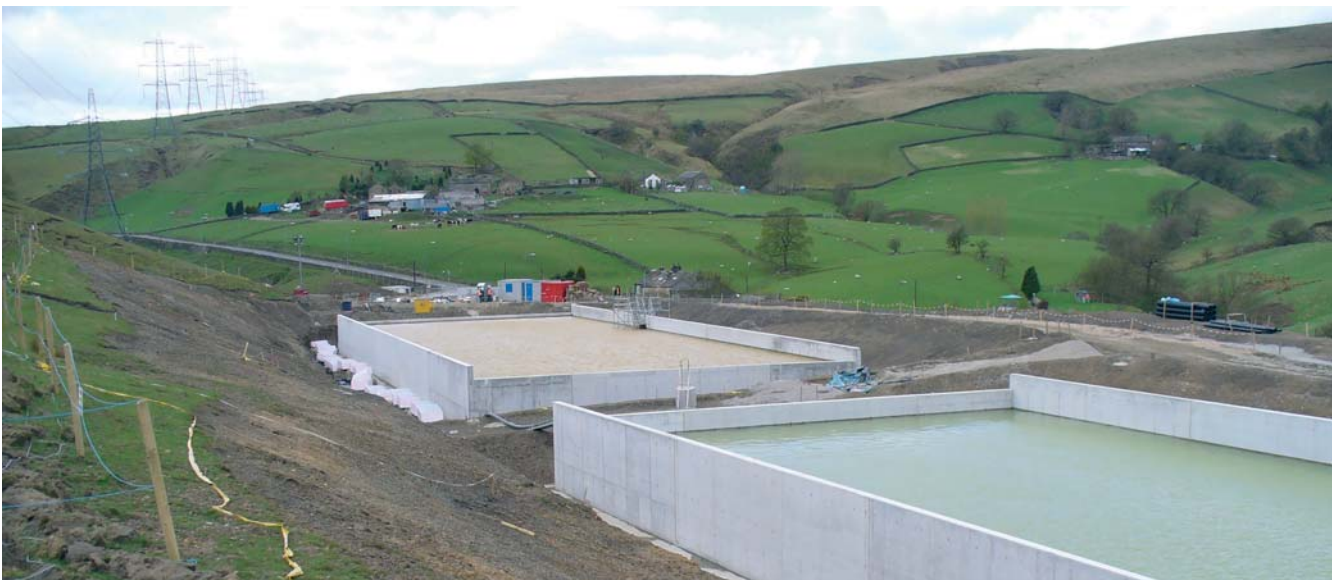
Completed lagoons during water test
