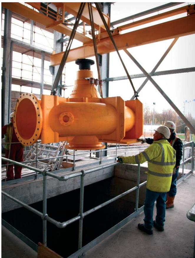
*The Belfast Sewers Project team begin to lower the pump into the shaft of the Terminal Pumping Station (TPS). The pump is one of 6 No. 15 tonne stormwater pumps which have been installed 40m below ground level at Duncrue Street, at the base of the project's TPS*
