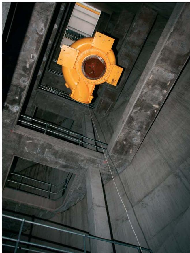
*The pump makes its way down the shaft, 40 meters below ground level. The pumps are crucial elements to the whole project and work to alleviate storm conditions and reduce the risk of flooding in the city*
